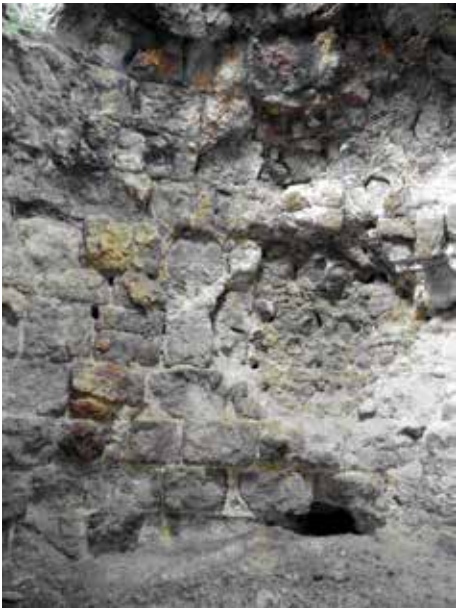
The side of the calcarone showing where the sulphur collected and was run out into moulds
