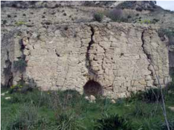
The side of the calcarone showing where the sulphur collected and was run out into moulds
