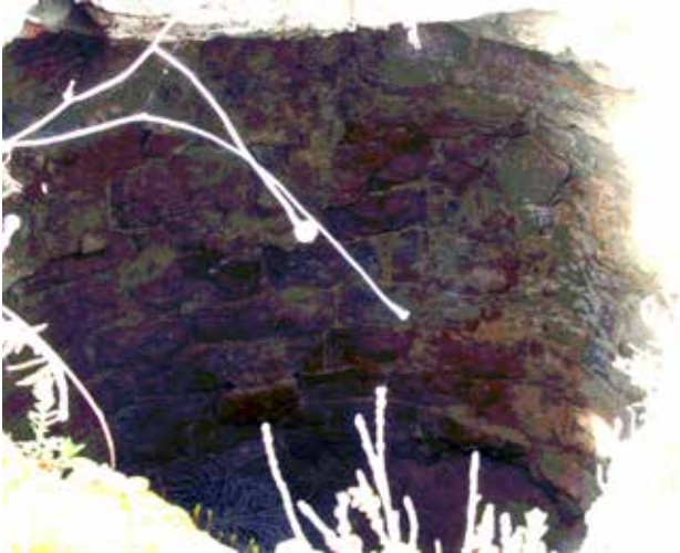
The inside of one of the four chambers – left from the top, on the right from below, the hole at the base is where the liquid sulphur ran out
